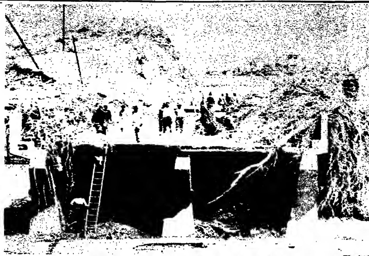
FLOOD HAVOC: Flash floods washed away this bridge outside the town of Laingsburg on the national highway between Cape Town and Johannesburg Monday. Sullen rivers and raging flood waters have left a trail of destruction throughout the Cape in which about 200 died or disappeared.
